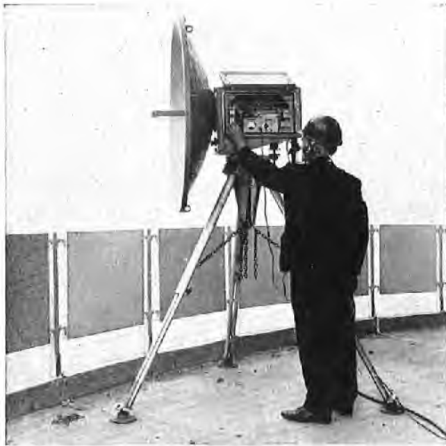
FIG. 12—TELEVISION OUTSIDE BROADCAST EQUIPMENT IN USE ON AERIAL GALLERY C1
