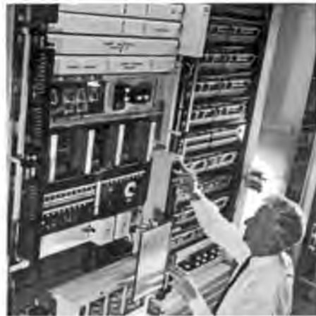
The charging rate for telephone calls is selected by means of switches which provide for cheap or full rate metering pulses according to a prearranged programme.
