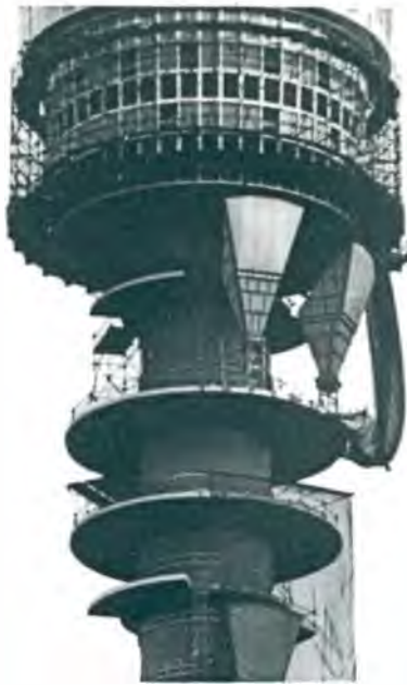
The first two giant aerials are fitted into position.
