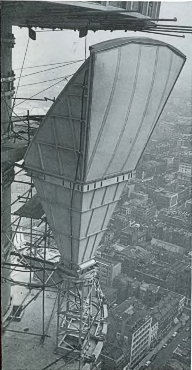
One of the horn aerials being fixed in position.
