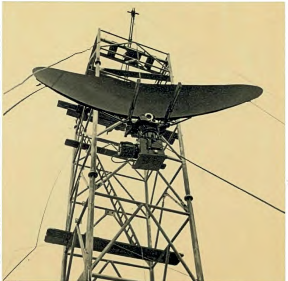
The aerial and turning gear of the Weather Radar being hoisted in position 620 feet above London. The radar will enable forecasters at the Holborn Weather Centre to see on display screens the position and extent of rain areas.
