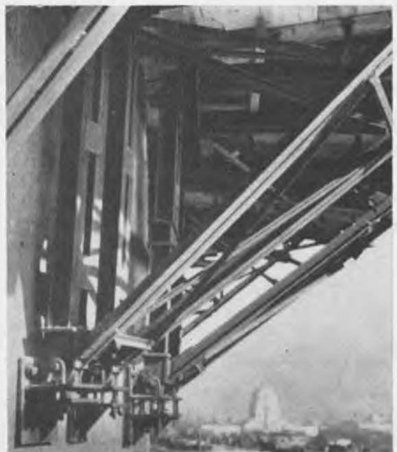
4 in units comprising timber frames. Eighteen units were decking fixed to two steel required for one floor
