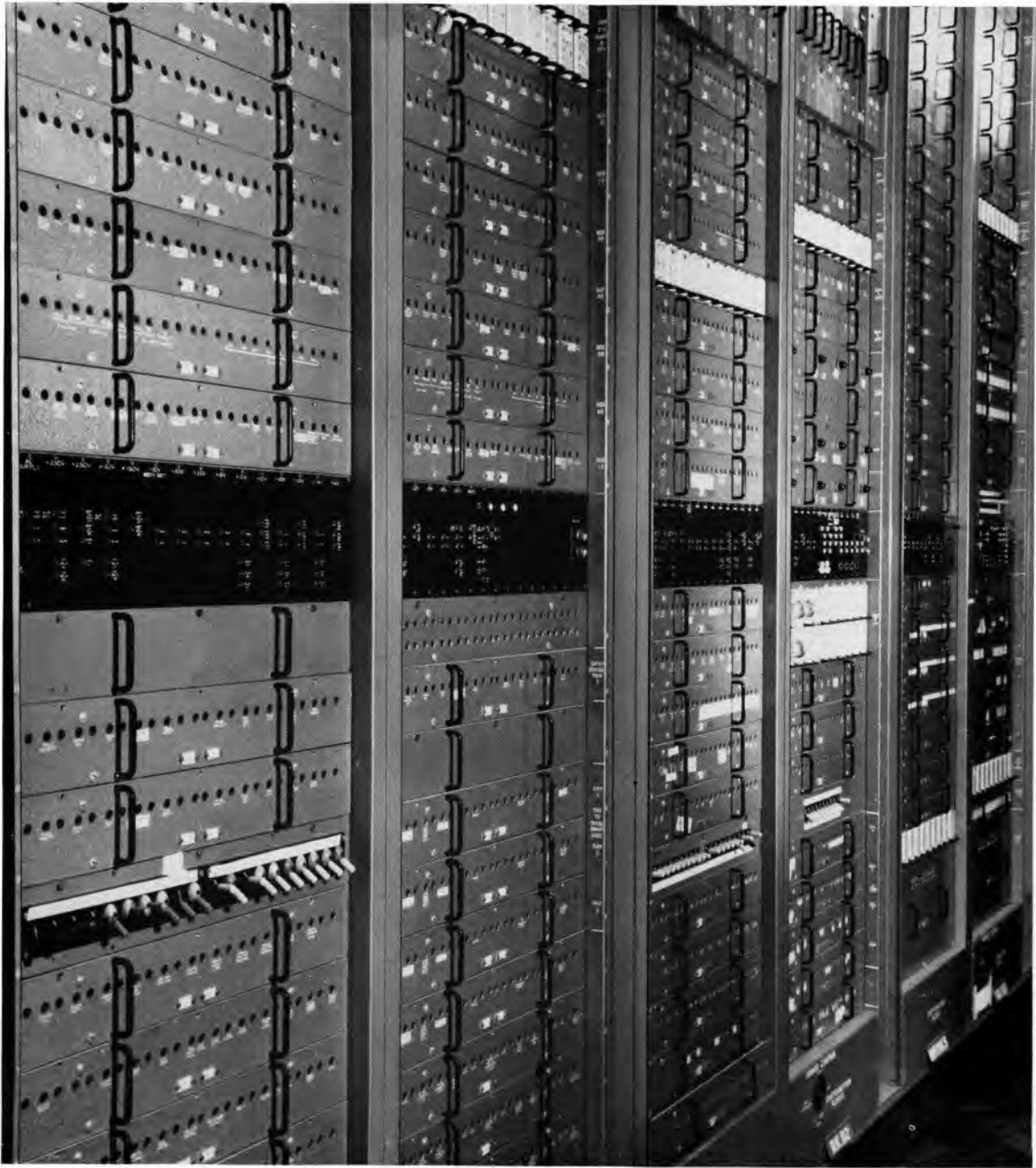
Frontispiece Time division multiplex suite in the electronic telephone exchange, Highgate Wood, North London.
