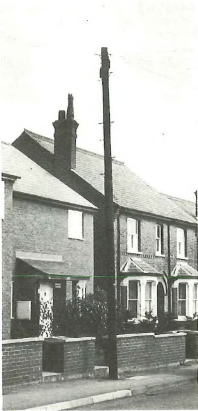
(a) A typical wood distribution pole
