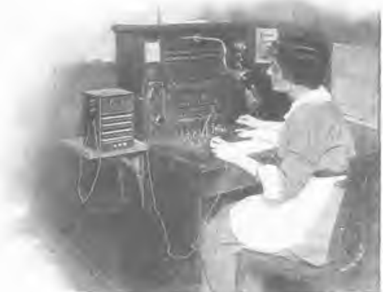
Dictograph Intercom at a Telephone Switchboard
