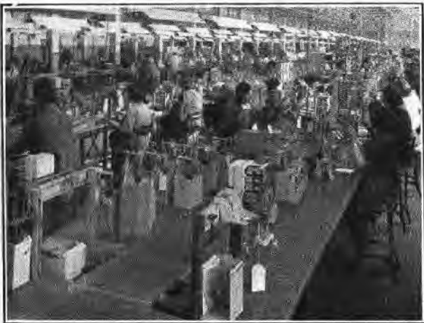
ASSEMBLY AND WIRING SHOP.
